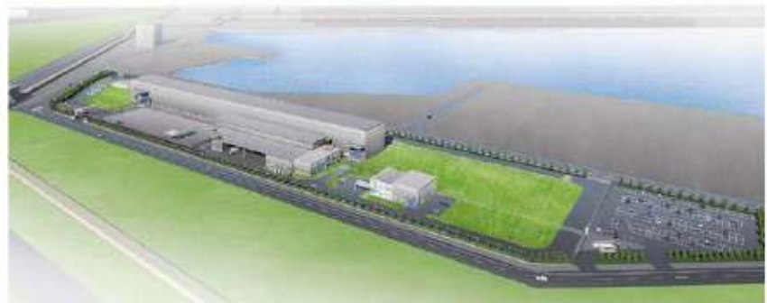
New Himeji Factory Scheduled to commence operation in October 2018
