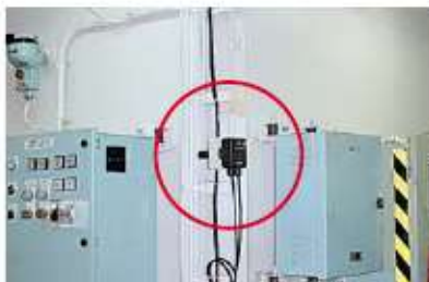
Beside rudder unit
