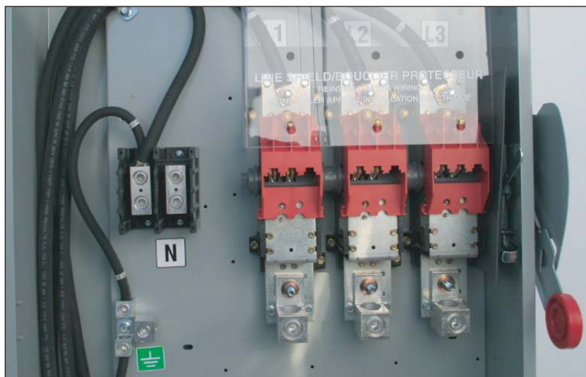
Figure 21 - Generator Output Connection Lugs
