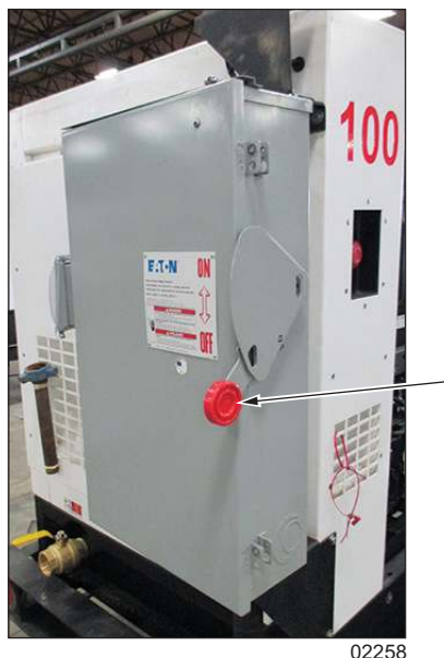
Figure 13 - Disconnect Lever
