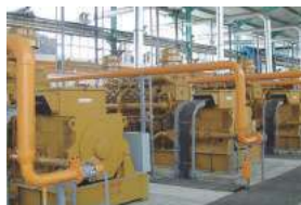
Sudan Natural Gas power plant Project
