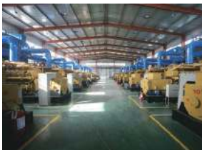
The coal mine gas genset power plant project in Shanxi
