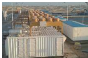
Niger Natural Gas Power Plant Project
