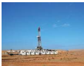
Gas engine drilling project in Karamay
