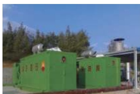
Biogas generator set power plant in Sichuan
