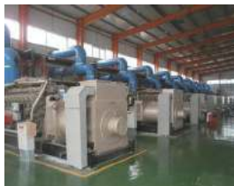
The coal mine gas genset power plant project in Shanxi
