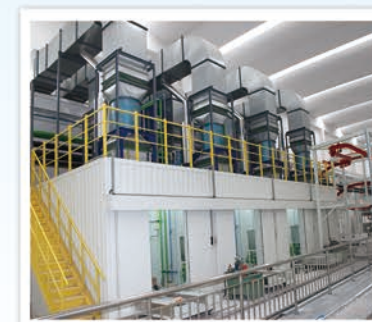
测试台架 Test bench
