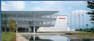
BIWA FACTORY ■ Vertical water-cooled diesel engine manufacturing ■ Vertical water-cooled gas engine manufacturing
